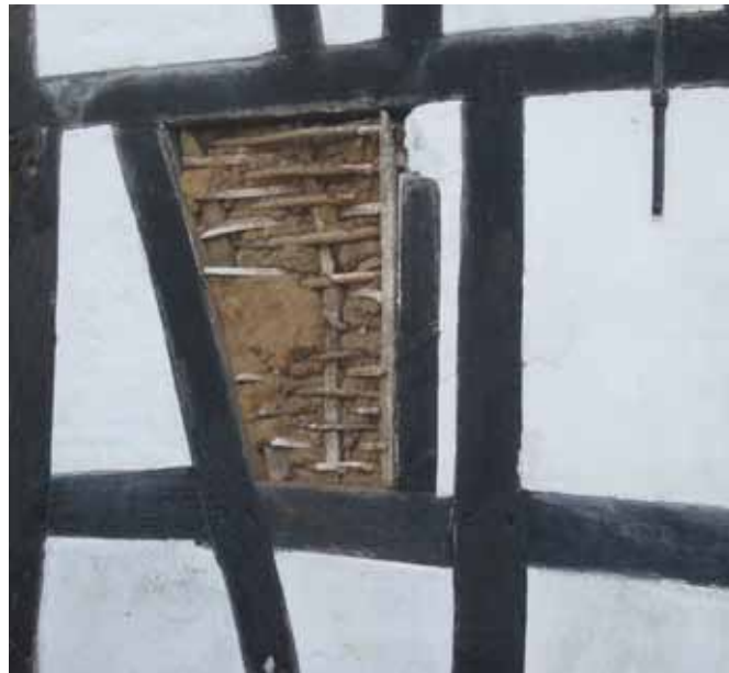
Walls made of wattle and daub Wikimedia Commons (CCL)
