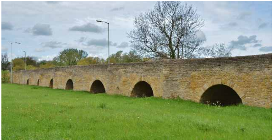
Bromham Bridge extends over a floodplain © Ashley Dace, Geograph (CCL)
